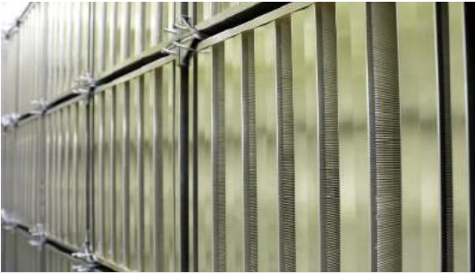
Highly-sealed HEPA installation
